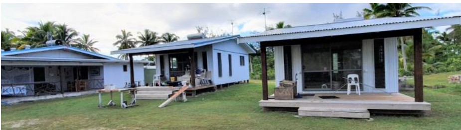
ONE BEDROOM VILLAS WHILE UNDER CONSTRUCTION — AWAITING NEW IMAGERY
